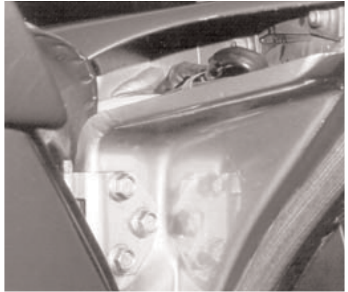
Remote location make the socket head screws challenging to loosen. Photo: M. Budinski
